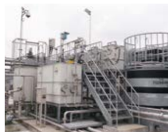
Wastewater treatment facility
