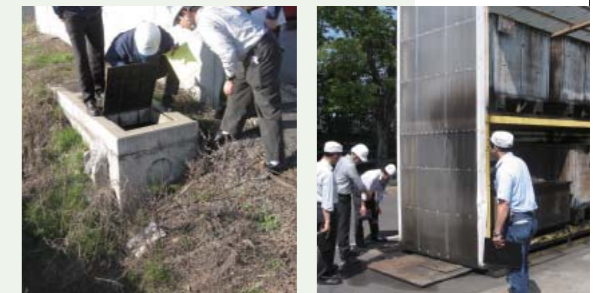
Examination of drain system
