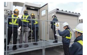
Drill to restore a primary power source
