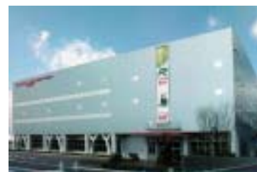
TOYOTA Material Handling Customer Center
