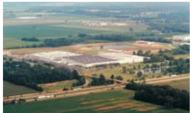
TIEM's plant in Columbus, Indiana
