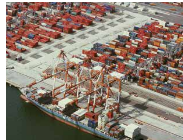
Tobishima Container Berth
