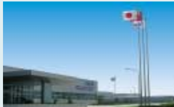
TD Automotive Compressor Kunshan Co., Ltd.
