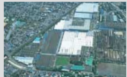
Kariya Plant develops and assembles compressors.
