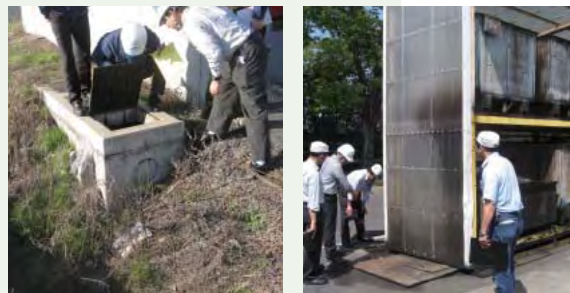
Examination of drain system
