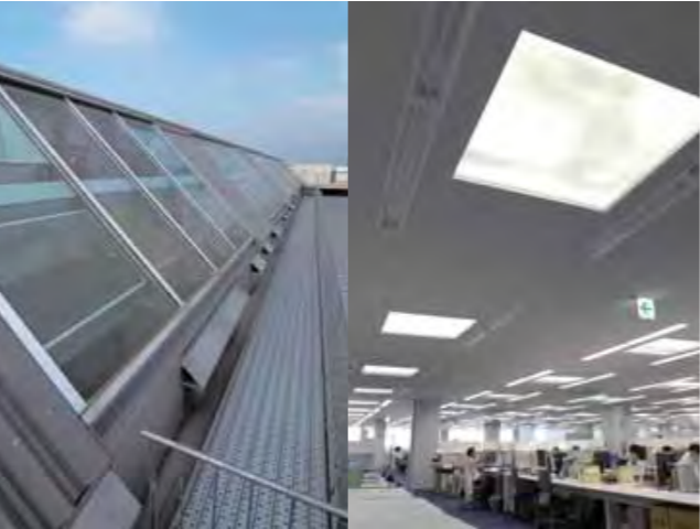
Light duct and light control system (Takahama Plant, Aichi Prefecture)
