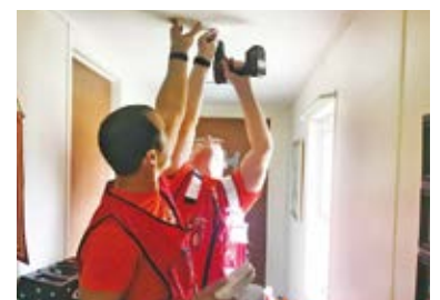
Inspecting a smoke alarm
