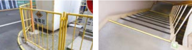
Hazard markings on uneven floors and stairs
