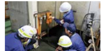
On-site inspection of detection performance
