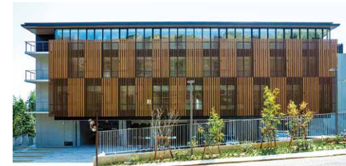
Company-built welfare facility
