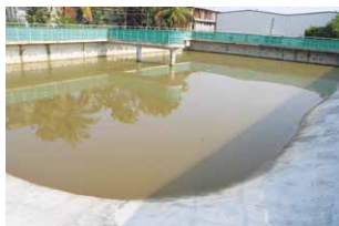
Pond for rainwater storage
