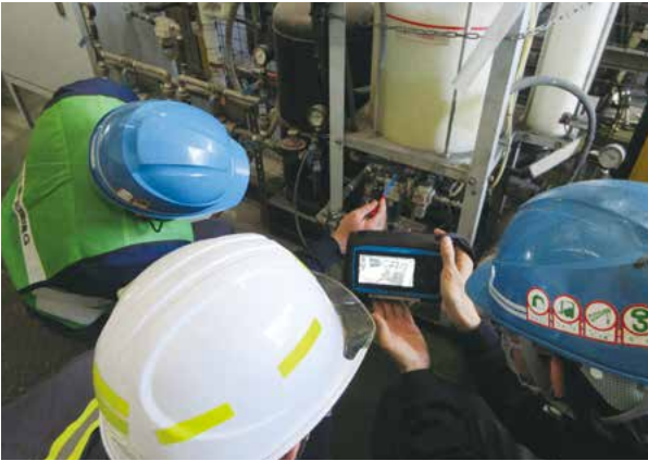
Observing air leakage using a camera
