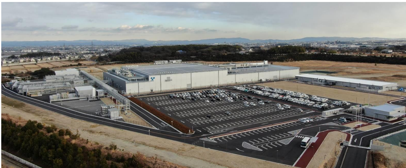
Ishihama Plant (Aichi prefecture)
