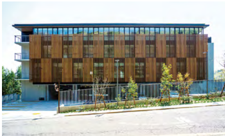
Company-built welfare facility
