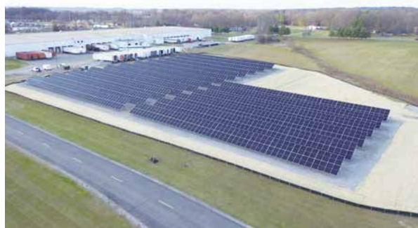
Solar panels installed on the idle land
