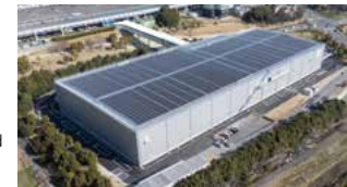
Newly constructed distribution center
