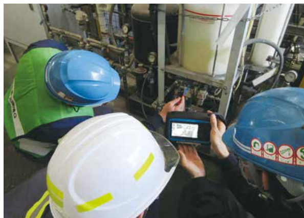
Observing air leakage using a camera
